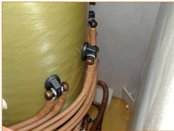
All the metallic surfaces of naked copper result covered by an adherent layer of black dust of  $Cu_2S$
